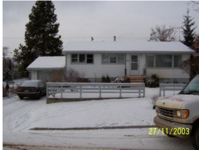
Overview of the Building
