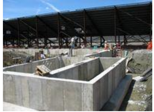
Poured Concrete - Crawl Space
