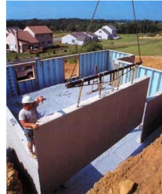
Poured Concrete Foundation Panels
