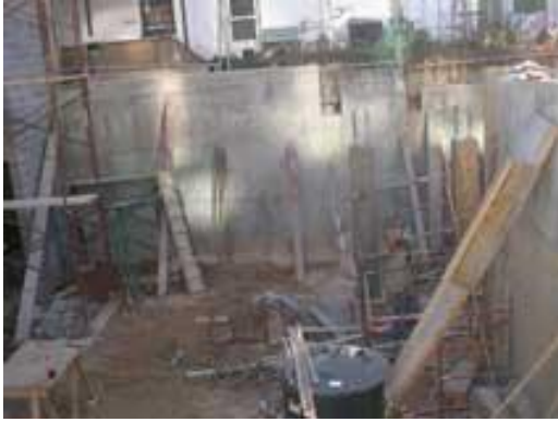
Poured Concrete - Full Foundation
