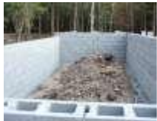
Concrete Block Foundation Wall
