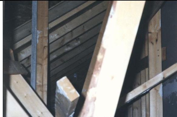
Photo 2 - Typical engineered truss system with long runs of 2 x 4 trusses.
