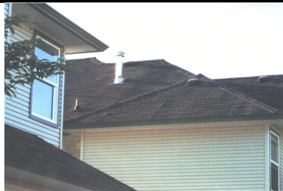
Photo 5 - Typical truss lines under composite roof shingles
