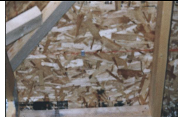
Photo 3 - Typical approved OBS (strand board) roof sheathing with H clips.
