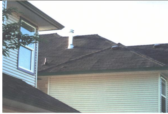
Photo 5 - Typical truss lines under composite roof shingles
